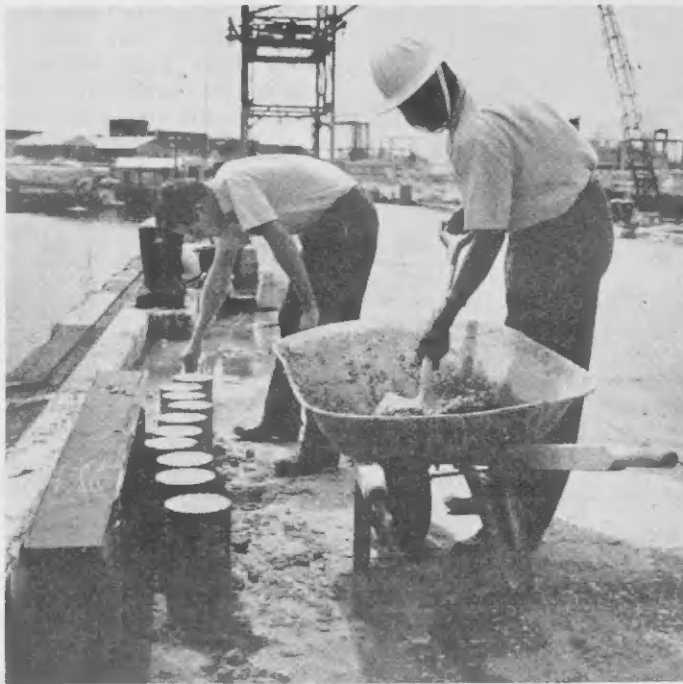
CORE SAMPLES were taken throughout the big pour. The hopper rider and vibrator man had unusual tasks.
